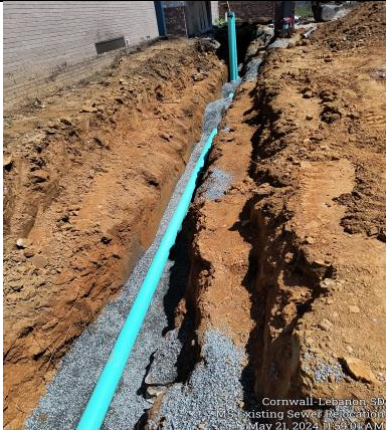
New Middle School Sewer Installation
