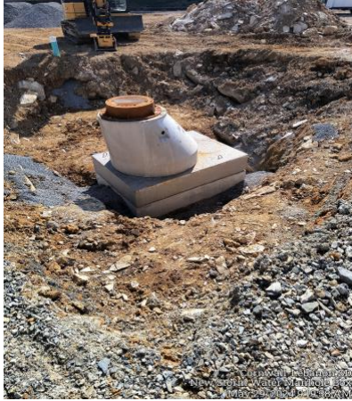
New Storm Water Manhole
