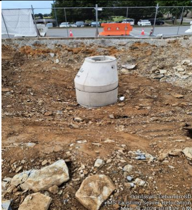
New Sewer Manhole on Building Pad
