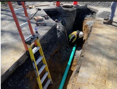
Force Main Connection at Monticello Drive
