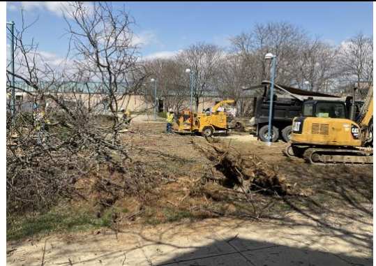
Tree Removal at Falcon Connector Site
