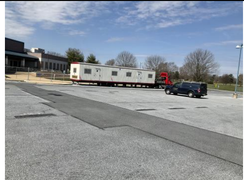
Arrival of Job Trailers
