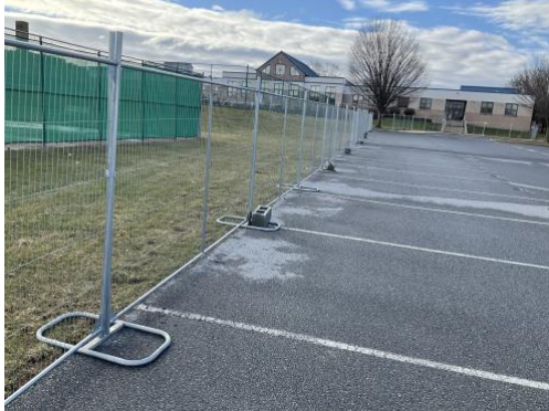
Installation of Security Fence
