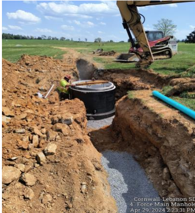
4" Force Main Manhole Installation
