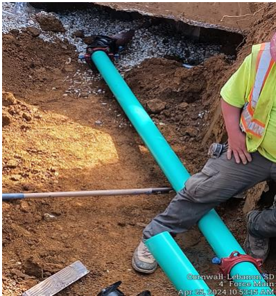
4" Force Main Connection To Pump Station
