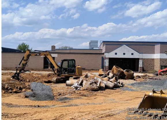
Storm Water Pipe Removal On Building Site Pad
