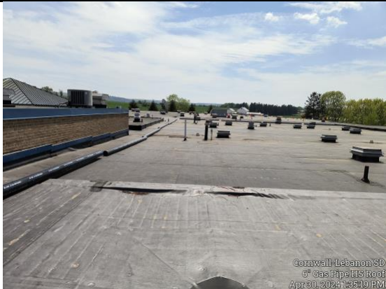
6" Gas Pipe Installation on HS Roof
