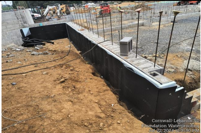
Foundation Waterproofing Installed
