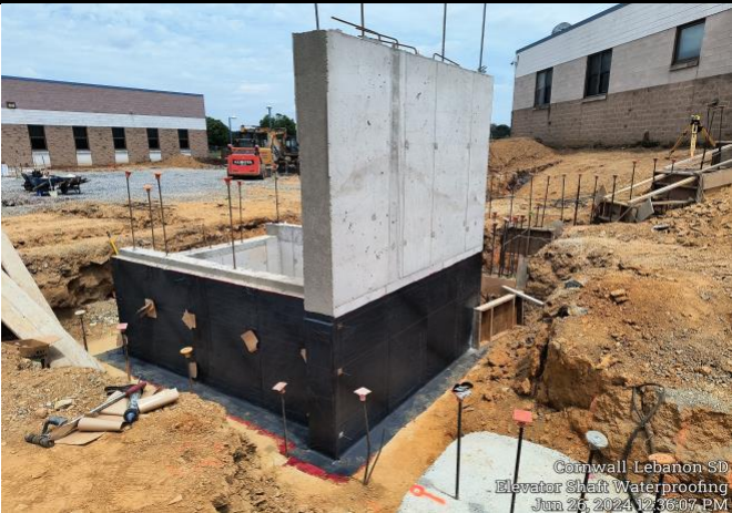
Elevator Shaft Wall and Pit with Waterproofing
