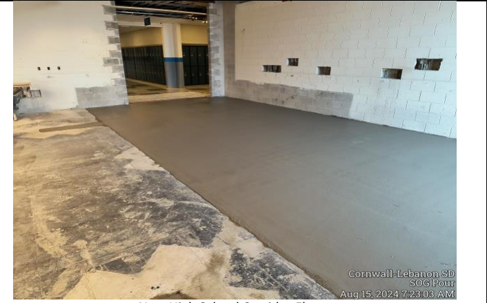
New High School Corridor Floor
