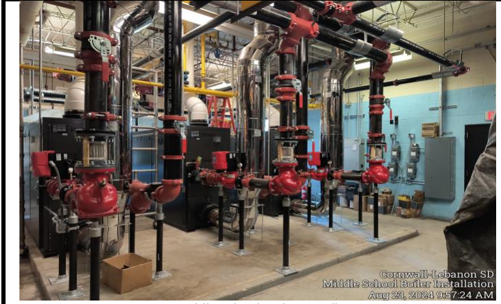
Middle School Boiler Install
