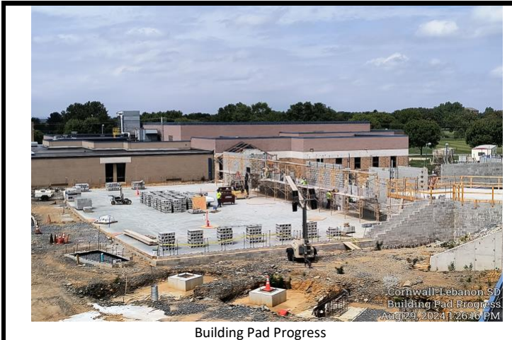
Building Pad Progress
