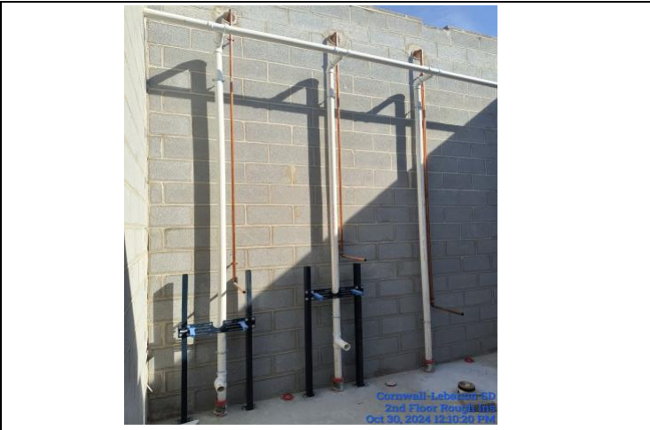
2nd Floor Plumbing Rough Ins
