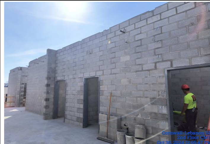
2nd Floor CMU Walls
