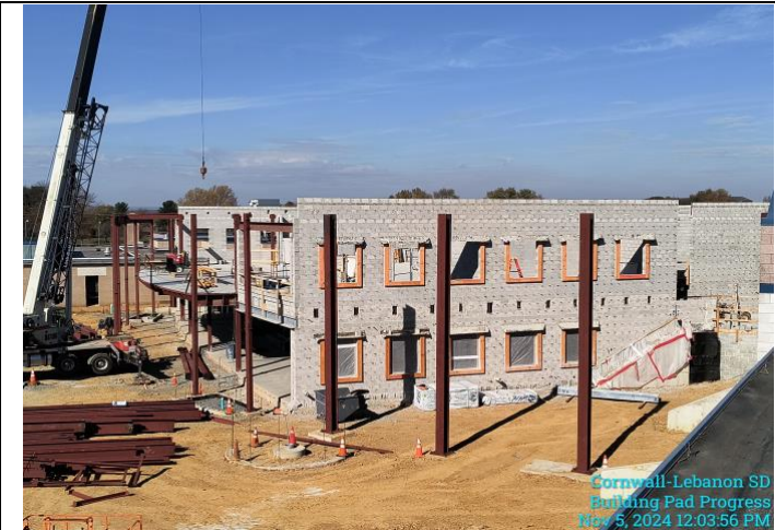
Building Pad Progress
