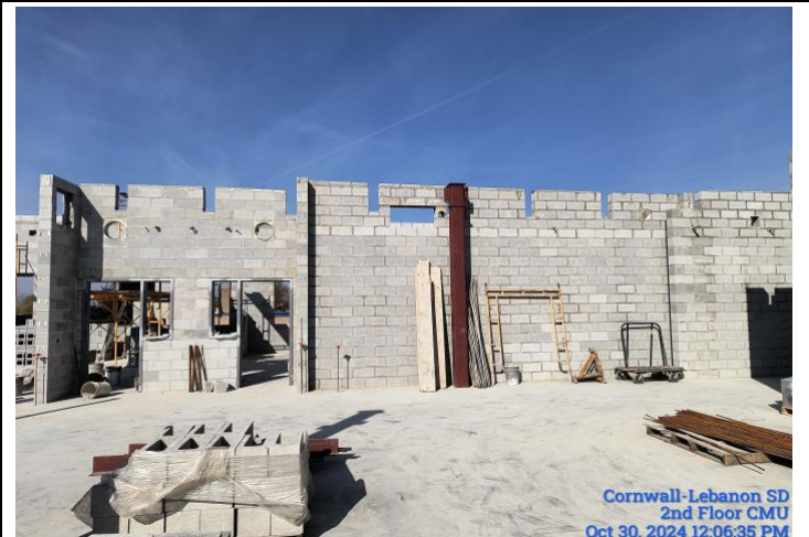
2nd Floor CMU Walls
