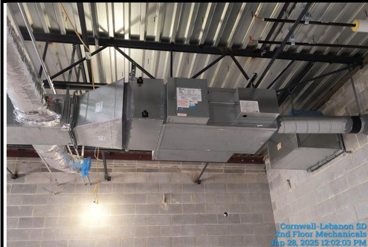
Ceiling Terminal Units Installed
