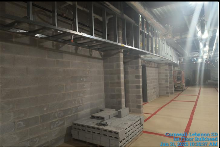
1 st Floor Radius Bulkhead
